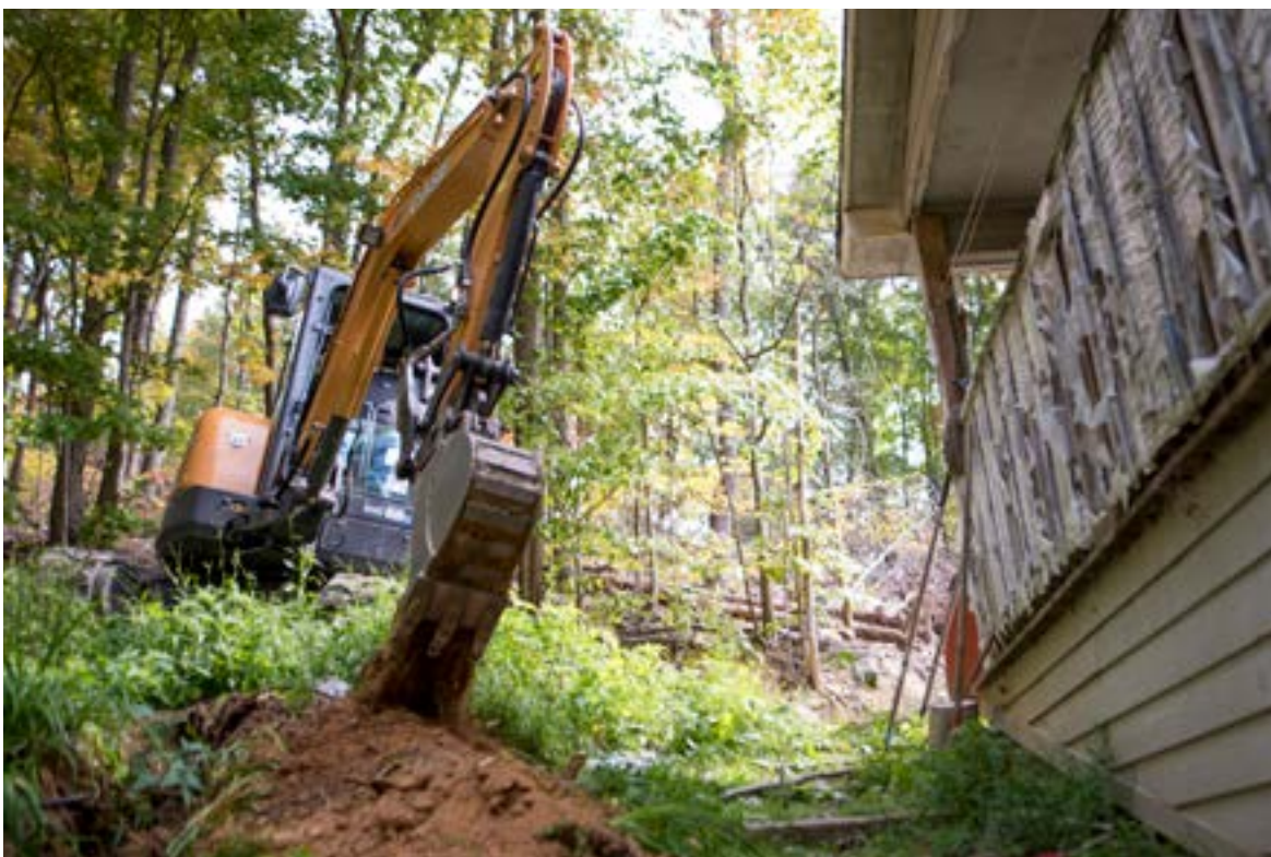
Appalachia Water Project installing a water line at a residence.
