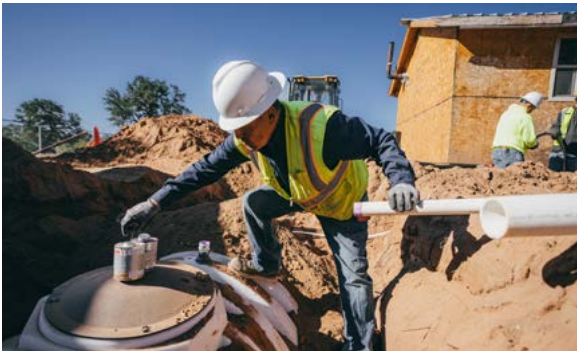
A DigDeep staff member installs a home water system for a homeowner in the Navajo Nation.
